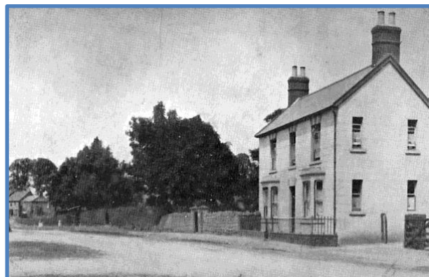
Photo above circa 1905. The old chapel stood in the middle of The Street by the trees and the road passed either side. (See Willington map on Key Page) The premises on the right was known as Lilemore Cottage. Both pictures above Courtesy of Paul Williams
