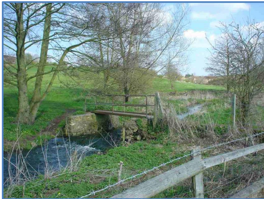
Above. The bridge over the dam walls.
