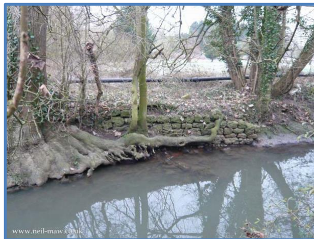
The wall blanking off the old mill channel cut at Watchfield House
